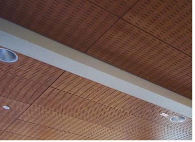
Flat Panel Series 7 (SS7) is available in standard and custom sizes to meet particular design requirements. Special surface patterns and logos can also be incorporated into the manufacture of the panels. Perforation options control sound absorption, and acoustic insulation is added behind panels for greater NRC performance. ACGI attaches acoustic fabric to the back of perforated panels to increase acoustical absorption.
