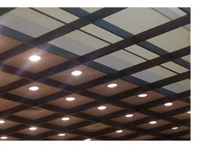
Continous Cube 2 (CC2) come in a variety of cell sizes, wood thicknesses and depths. Depending on project requirements, Cube panels can be factory or field-cut to size. Fixture cut-outs can be factory cut, but are typically cut to field conditions.
