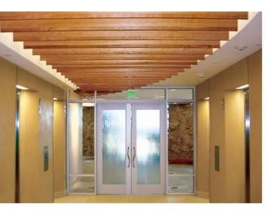
**Tremolo<sup>™</sup>** (TB1) is a tapered wood baffle that furnishes a stunning and impressive appearance. Each member suspends individually by HD T-Grid. An integral light fixture can be incorporated. Tremolo<sup>™</sup> baffles typically have a depth of 81/2", and can be manufactured in a wide variety of veneer.
