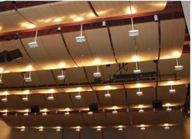
Allegro<sup>™</sup> Series 1 (AL1) provides a pre-engineered, pre-finished curved wood ceiling that easily suspends from a Unistrut<sup>®</sup> framing system. They are available in concave, convex or serpentine surfaces to meet both the acoustic and aesthetic requirements of the project. Panels suspend with a simple hanger system that provides security and accessibility. The panels are typically grouped together to form ceiling clouds. Allegro panels can also attach to walls.
